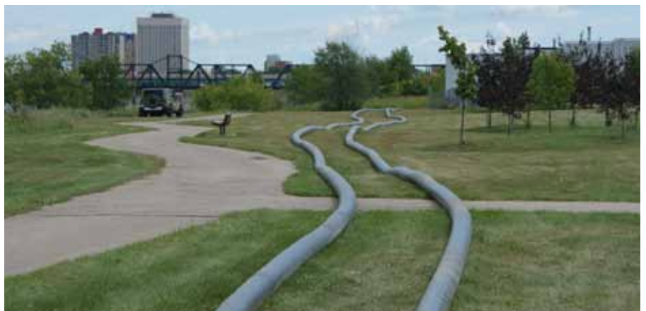
Pipes bringing water from the West Hill storm retention pond
