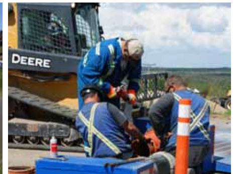
Assembling the temporary pipeline from the South Saskatchewan River
