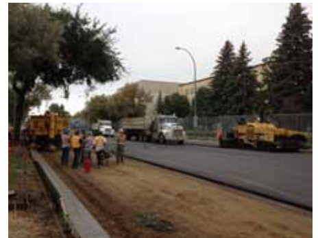
15th Street West paving
