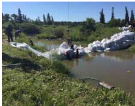
Pipes bringing water from the West Hill storm retention pond
