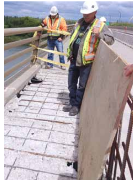
Diefenbaker Bridge restorations
