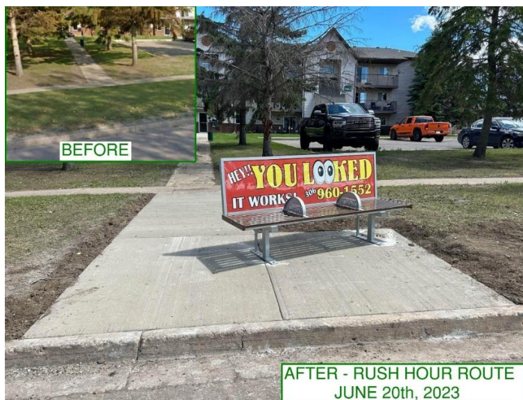
Figure 4: Example of new concrete transit pad with enhanced connectivity
