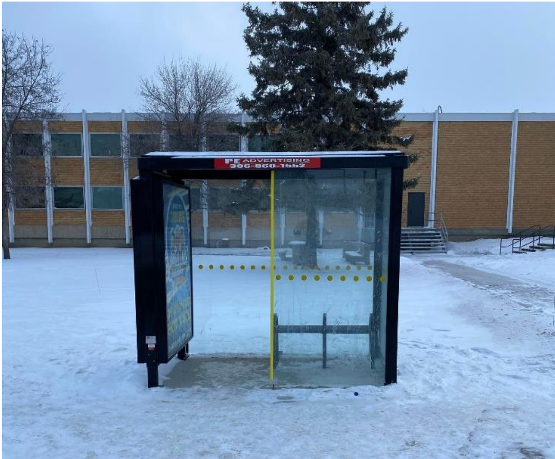
Figure 2: Carlton West Transit Shelter Installation
