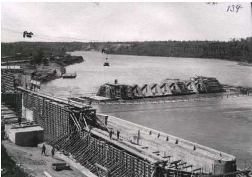
Looking west, upstream.
