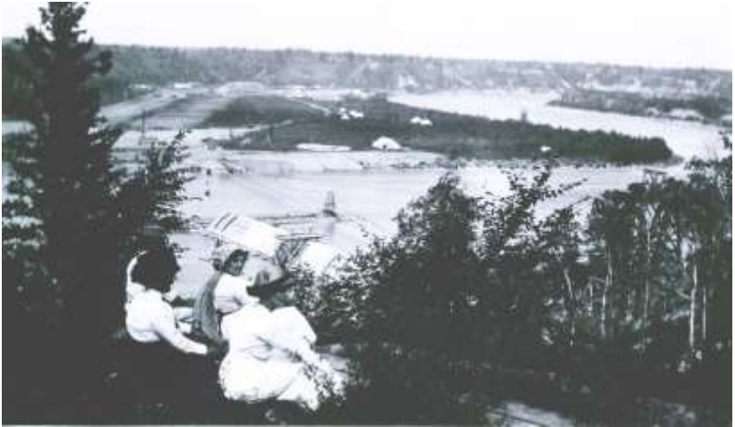
Summer entertainment watching the construction.
