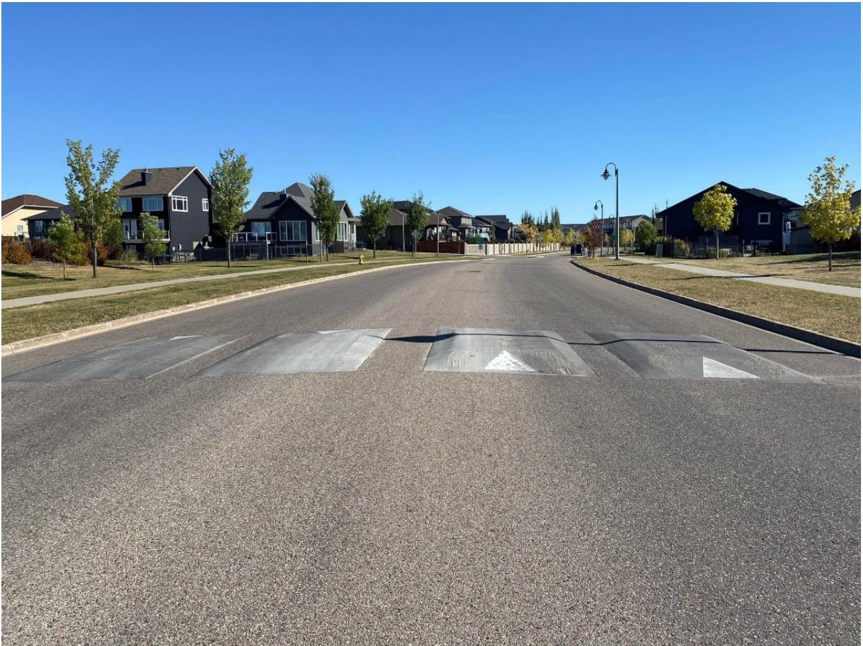
Figure 1: Vic Boulevard, Saskatoon Permanent Speed Cushion
