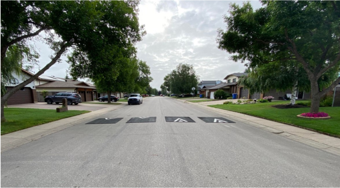
Figure 1: Temporary Speed Cushion – Barton Drive
