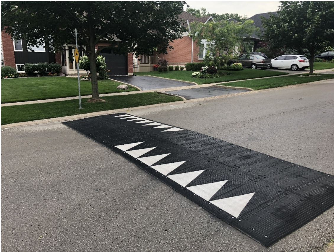
Figure 2: Temporary Speed Hump Example
