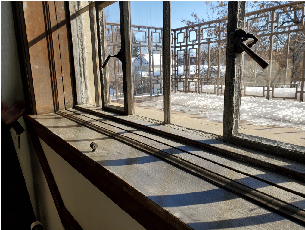
Figure 17 – Interior of steel 'T' frame rose window
