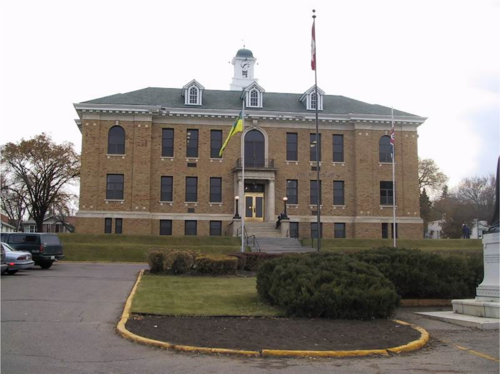
Figure 1 North main entrance façade – prior to window replacement
