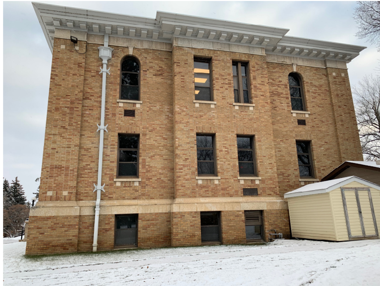
Figure 5 – West façade – close up – prior to window replacement
