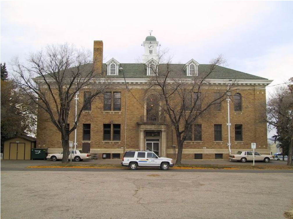
Figure 2 South façade – prior to window replacement
