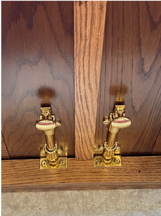
Figure 30 - 31 hardware – inside of new balcony doors
