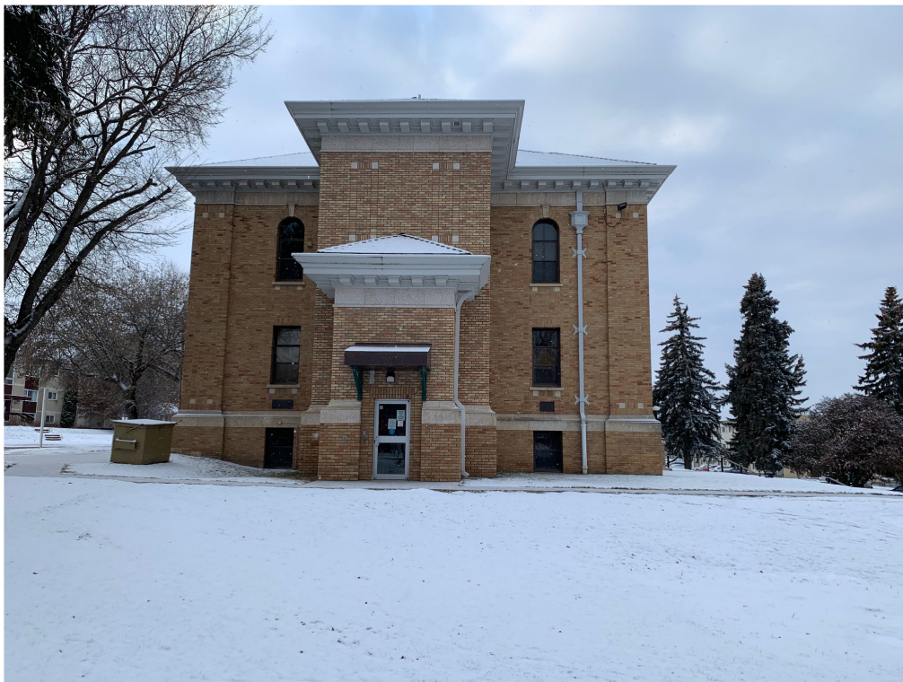
Figure 4 – East façade – present day with accessibility addition – prior to window replacement
