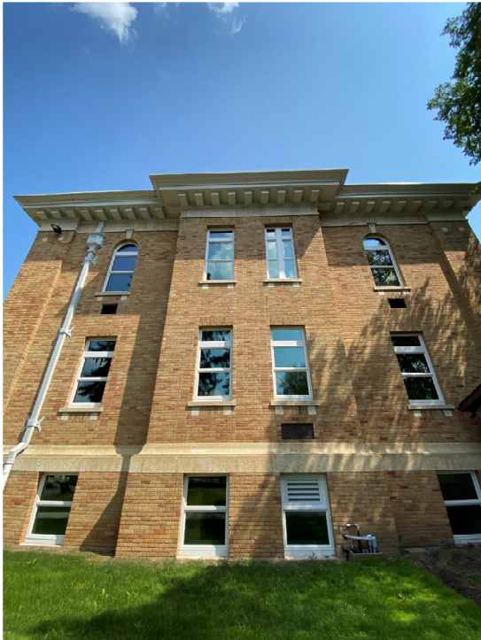
Figure 24 – West façade – new windows
