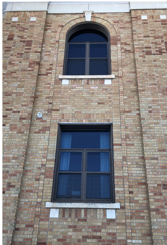
Figure 8 – Brick and stone detailing at window openings – prior to window replacement .
