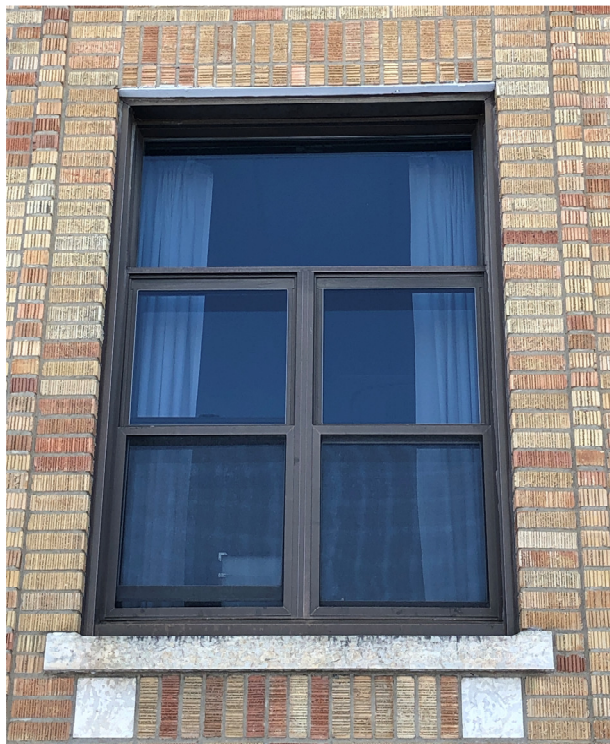
Figure 13 – Example of non-original aluminum windows – prior to window replacement Note how far back in the wall plane these windows are located.
