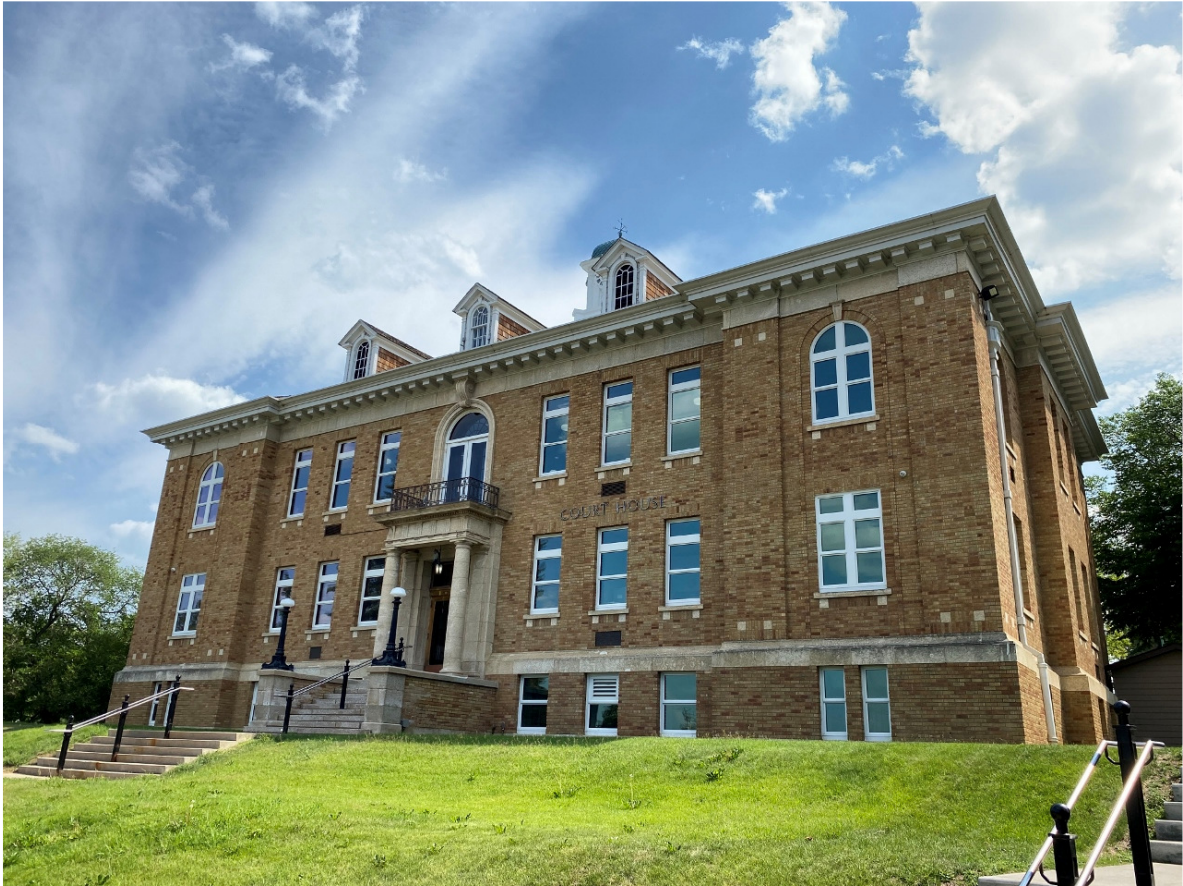
Figure 35 Main façade north – new windows
