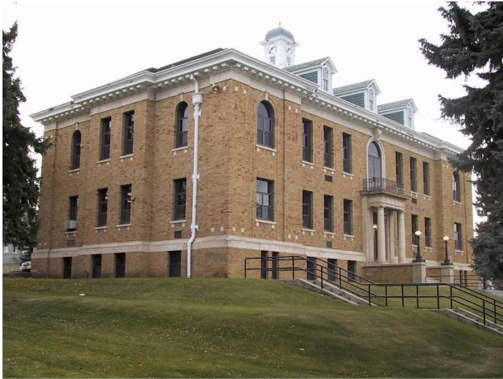
Figure 3 – East façade prior to accessibility addition and window replacement.
