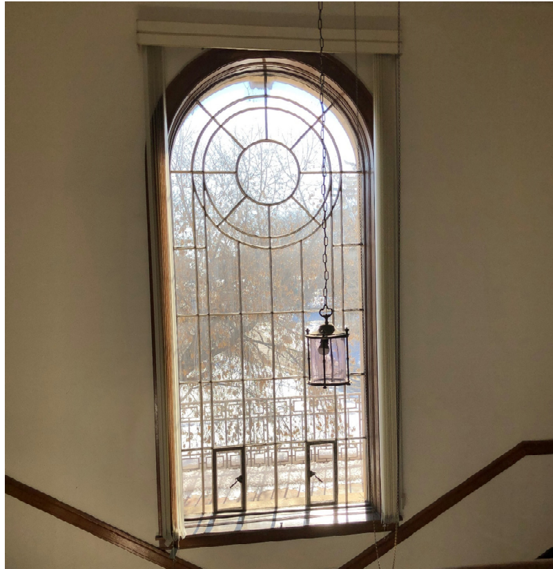
Figure 11 – Original steel 'T' frame rose window on south façade
