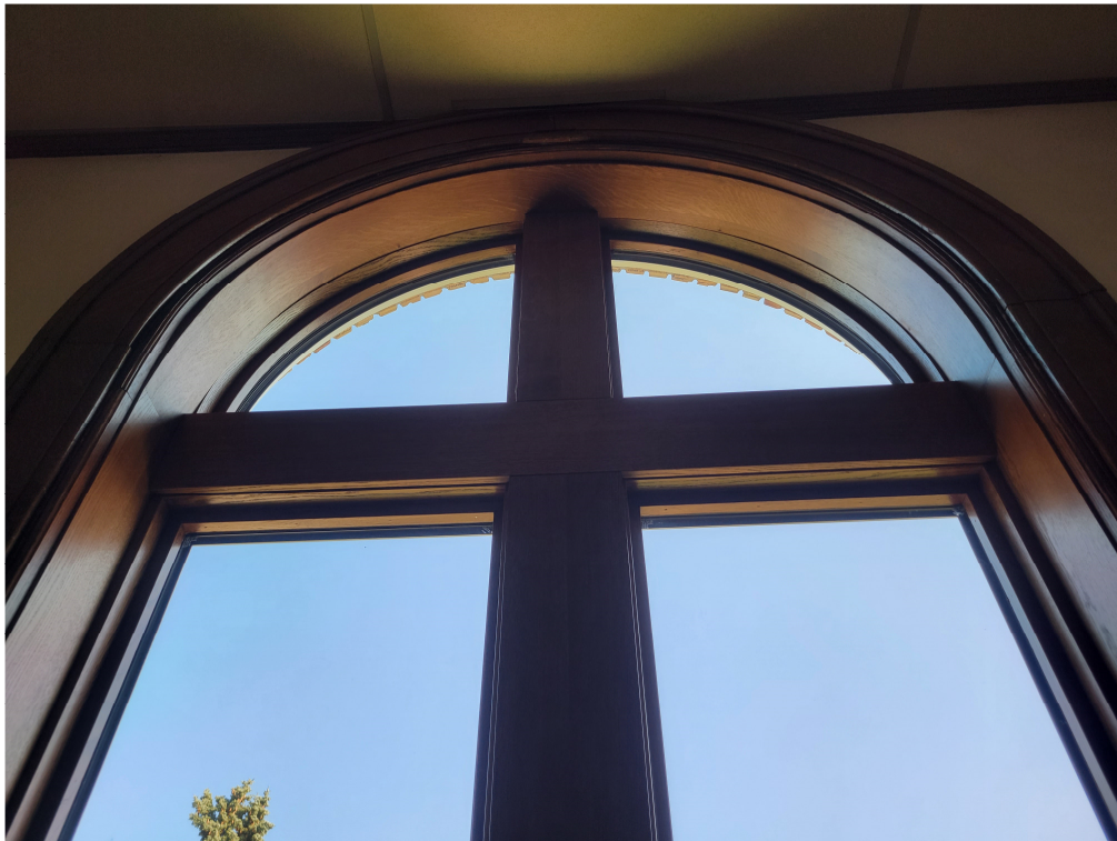
Figure 28 Interior arched windows – new windows
