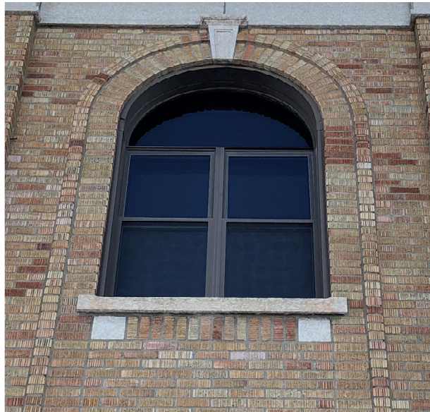
Figure 13 – Example of non-original aluminum windows – prior to window replacement Note how far back in the wall plane these windows are located.
