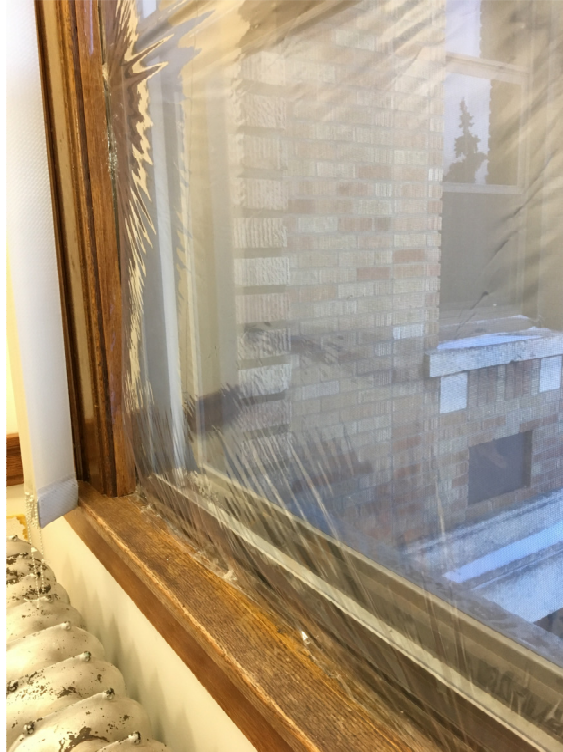
Figure 15 – window opening covered by plastic film to prevent air infiltration
