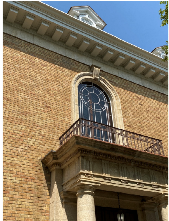
from exterior – new windows
