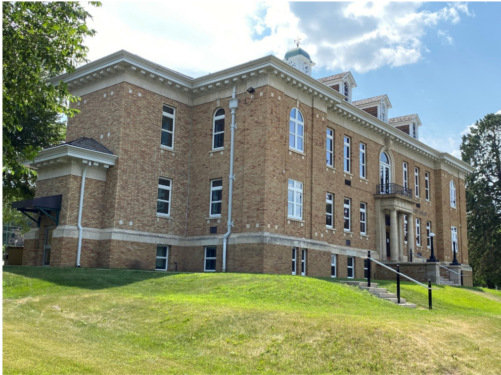
Figure 23 – East façade - new windows.
