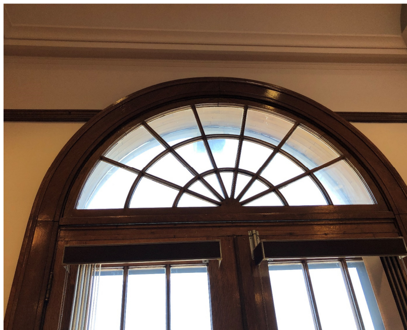
Figure 12 – Original wood fan arch window above oak doors on north façade above main entrance portico
