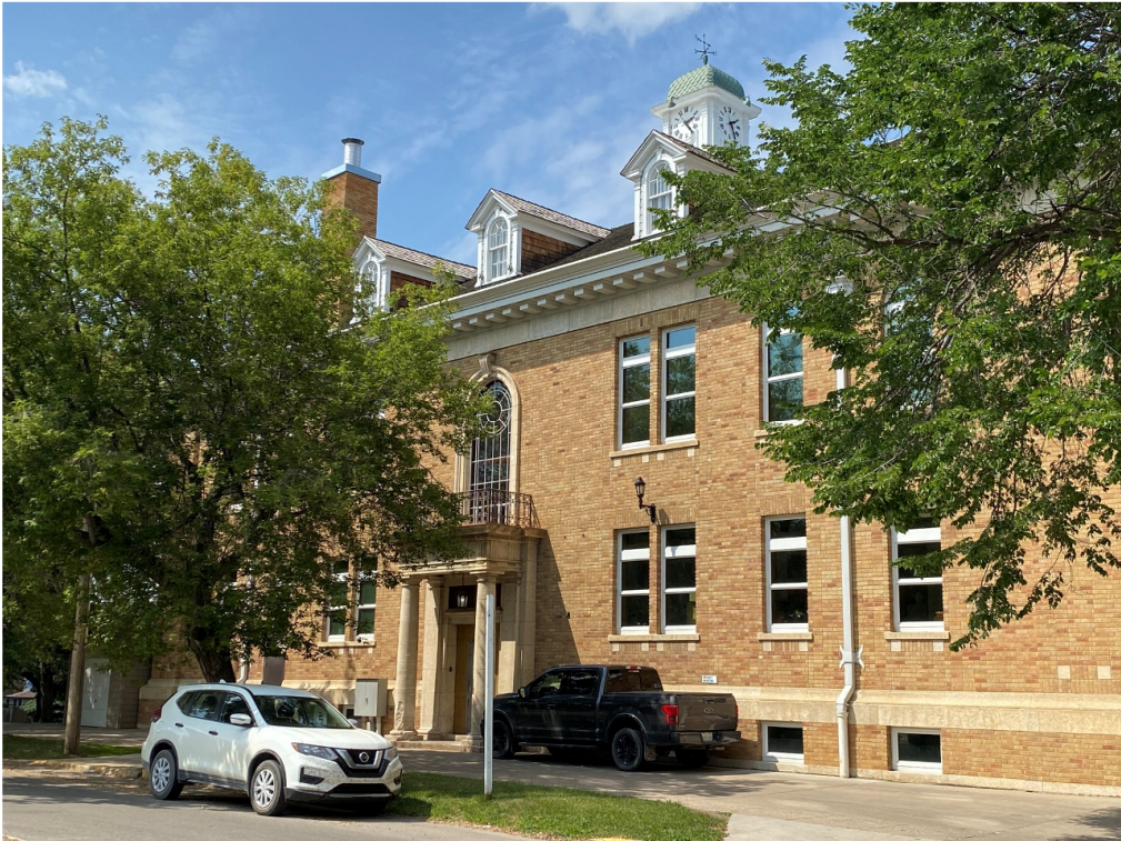
Figure 22 South façade – new windows
