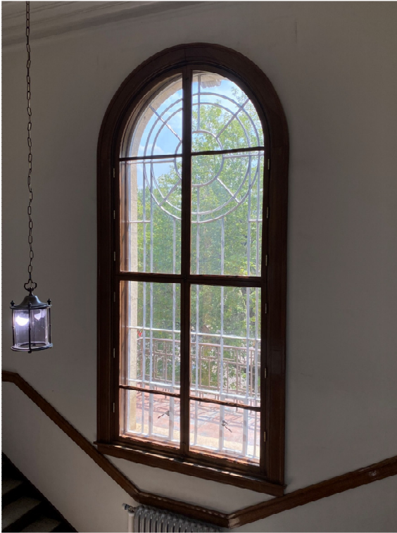
Figure 26 - 27 Rose Window from stairwell – new windows
