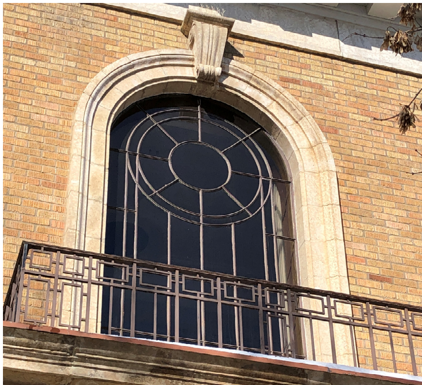
Figure 18 – Exterior view of rose window on south façade
