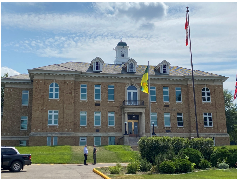
Figure 21 North main entrance façade – new windows
