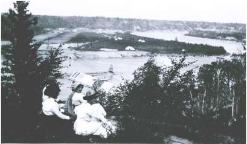
Summer entertainment watching the construction.
