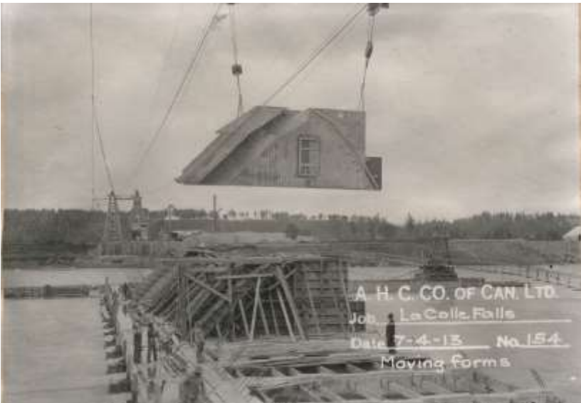
The towers and cables for heavy lifting.
